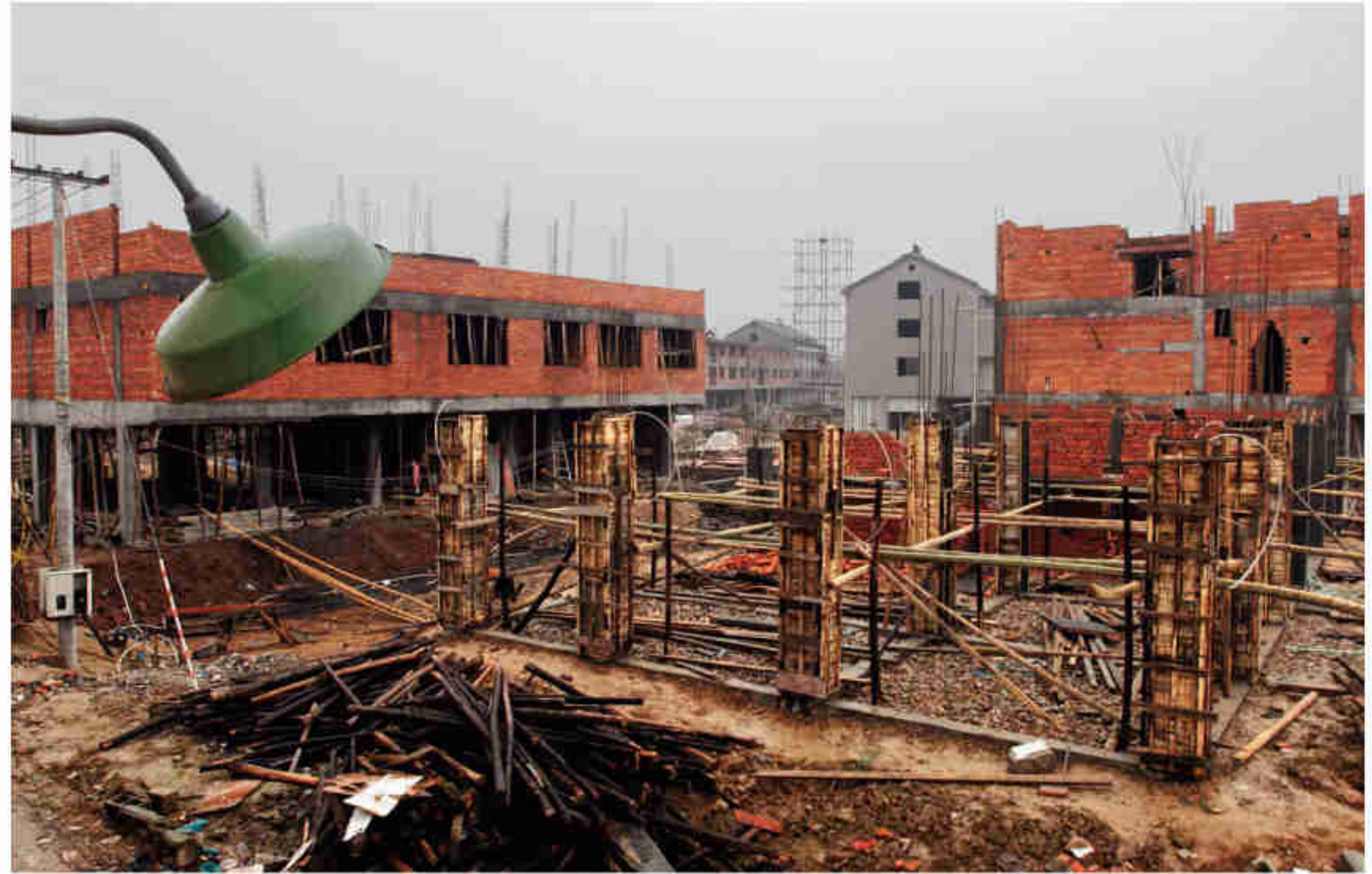
DECEMBER 2005: LOWER FLOORS
